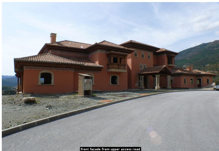
front facade from upper access road
